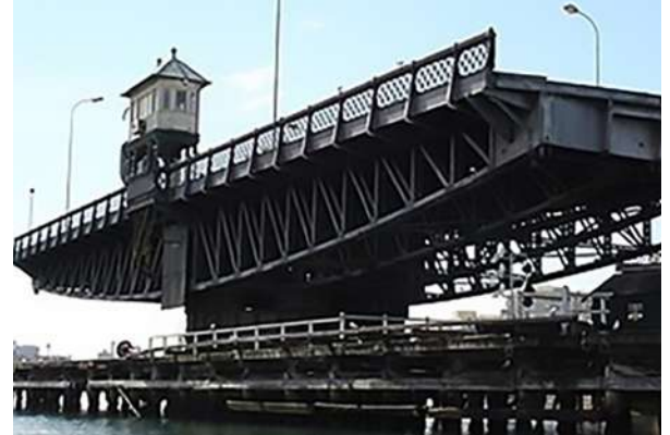
The elevation of the Glebe Island Bridge showing pivot, rest and buttment piers, as well as the delightfully curved central swing span.
